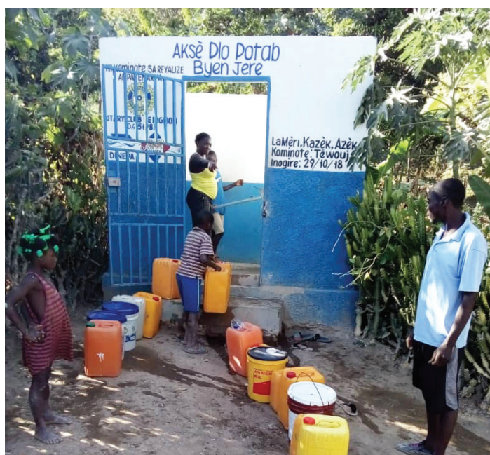
New community well—closer, safer way to get clean water.
